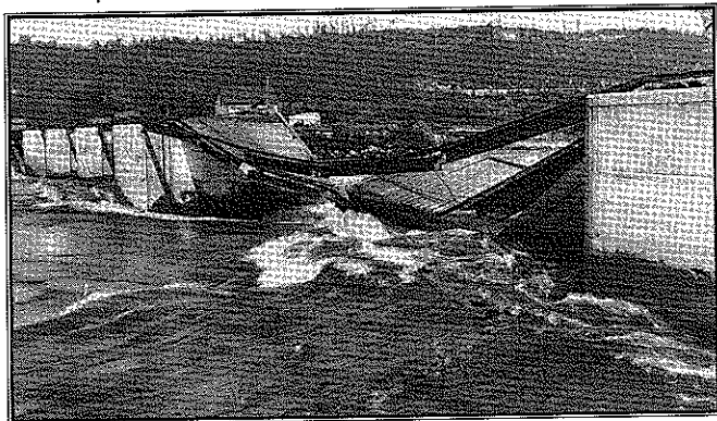
Collapse of the dam.
