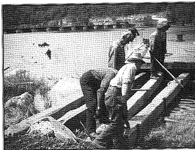
July 1938 - building a landing for the ferry which will take cars across Lake Temiscaming while repairs are made on the Ontario dam.
