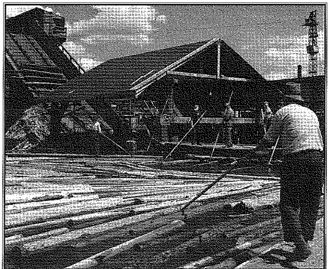
Employees at work at the foot of the jack-ladder.
