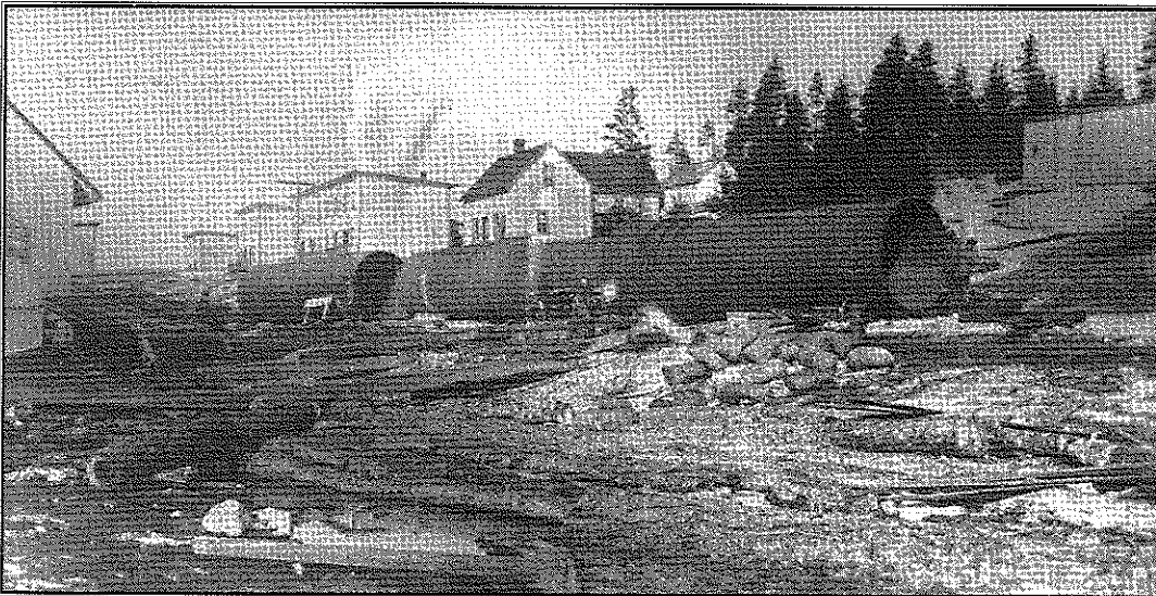
Construction of a pipeline.
