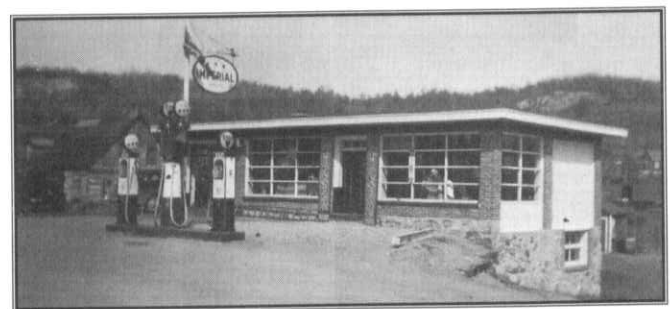
Esso garage has "new" gas pumps.
