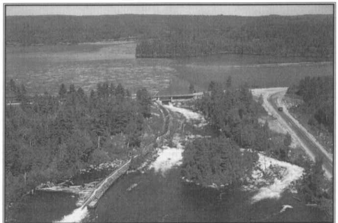
Log boom and timber slide in the Temiscaming and Kipawa area.
